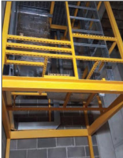
Figure 22: Prefabricated modules integrated with catwalk (Photograph courtesy of Laing O'Rourke)
