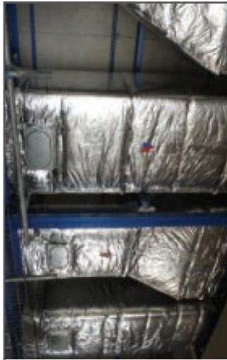
Figure 23: Riser with platform modules (Photograph courtesy of Balfour Beatty PLC)
